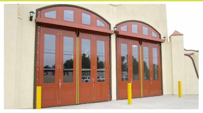
Door Engineering introduces their new Four-Fold XT<sup>™</sup>. Limited space in the apparatus bay can be concerning, but with Door Engineering's new inside-out design it is no longer an issue. The Four-Fold XT<sup>™</sup> operator is interior mounted while the door panels fold to the exterior. This eliminates the bay space that is needed with the regular Four-Fold design.
