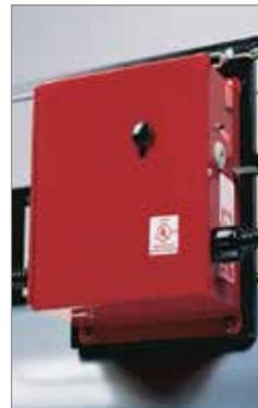
This device controls the release of the door in a fire emergency and provides protection for both people and property.
